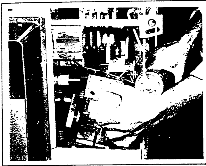
Fig. 32. Motor operator removal
