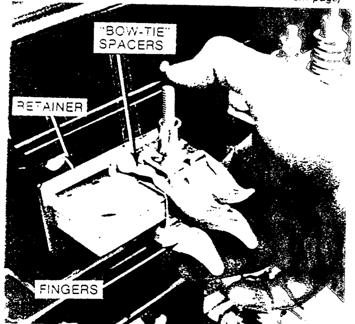
Fig. 45. Partial primary disconnect ASM
